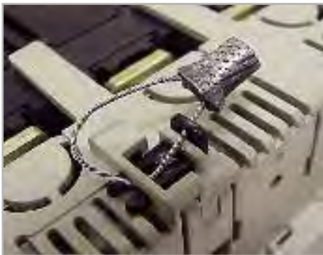
Terminal Cover Lock with Lead Seal
